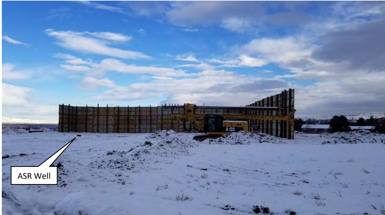
A sounds wall stands around the ASR well site.
