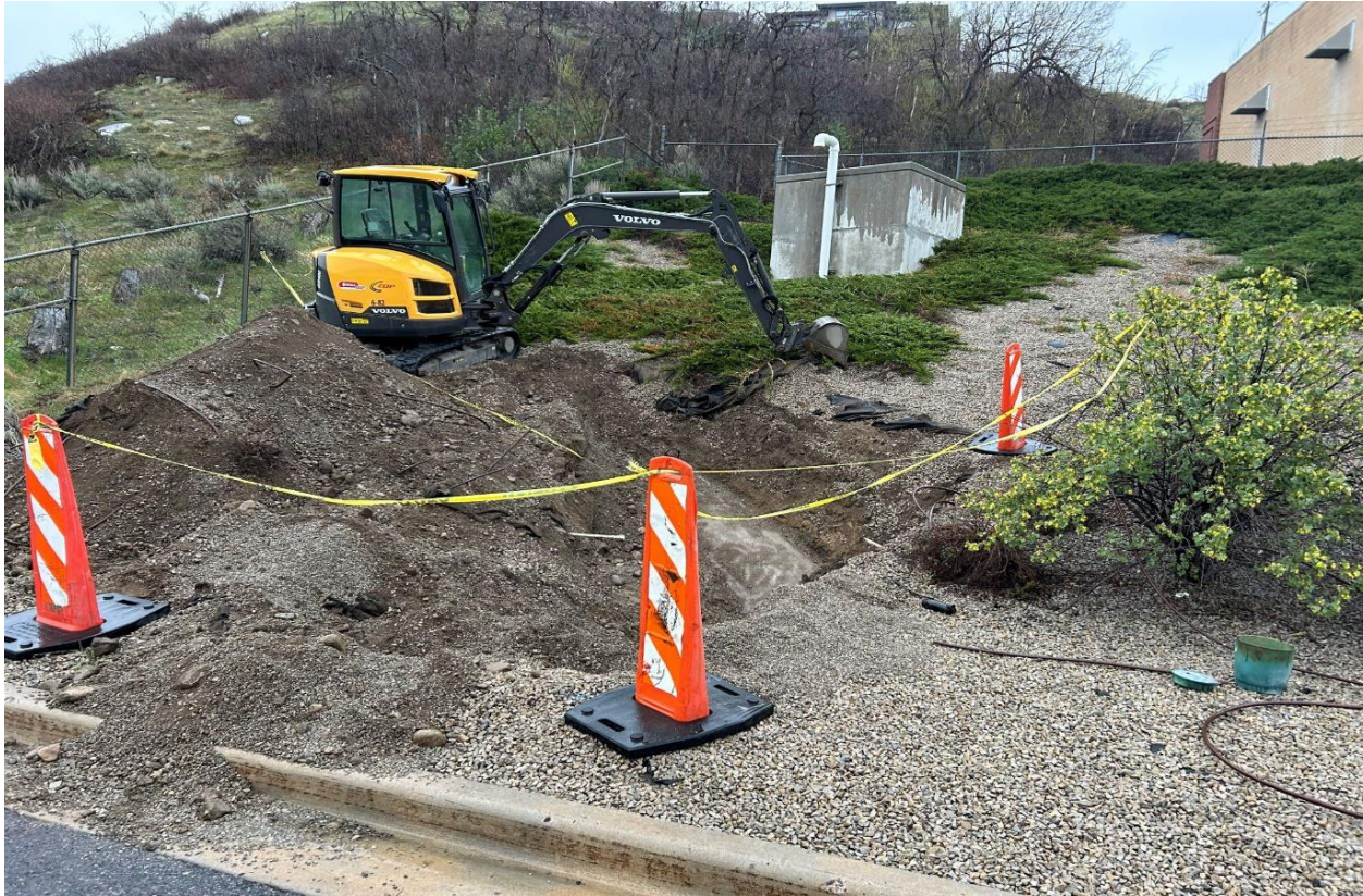
April 12, 2024: Potholing west of the Murray Power Plant.
