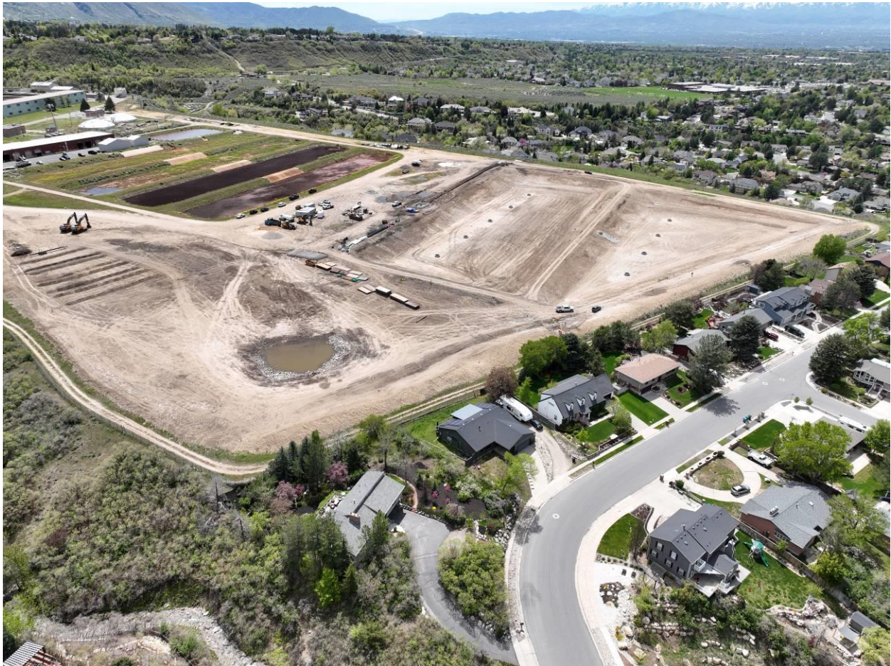
April 30, 2024: Overall site progress.
