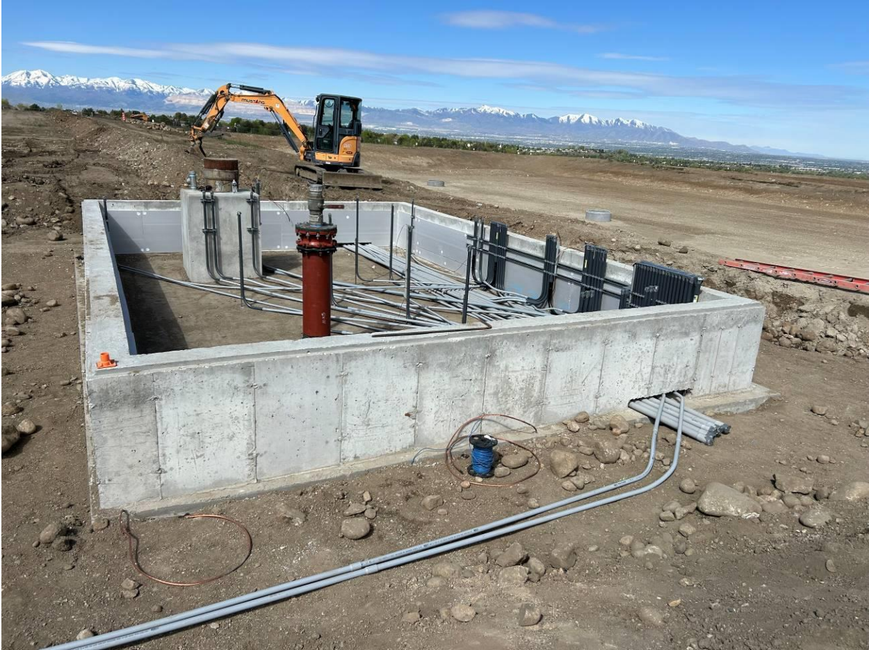
May 2, 2024: The well house foundation and conduits are in progress.
