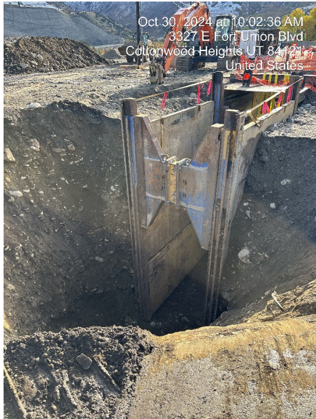
October 28 and 30: Excavating and pipe installation for the CC-1 vault is underway.
