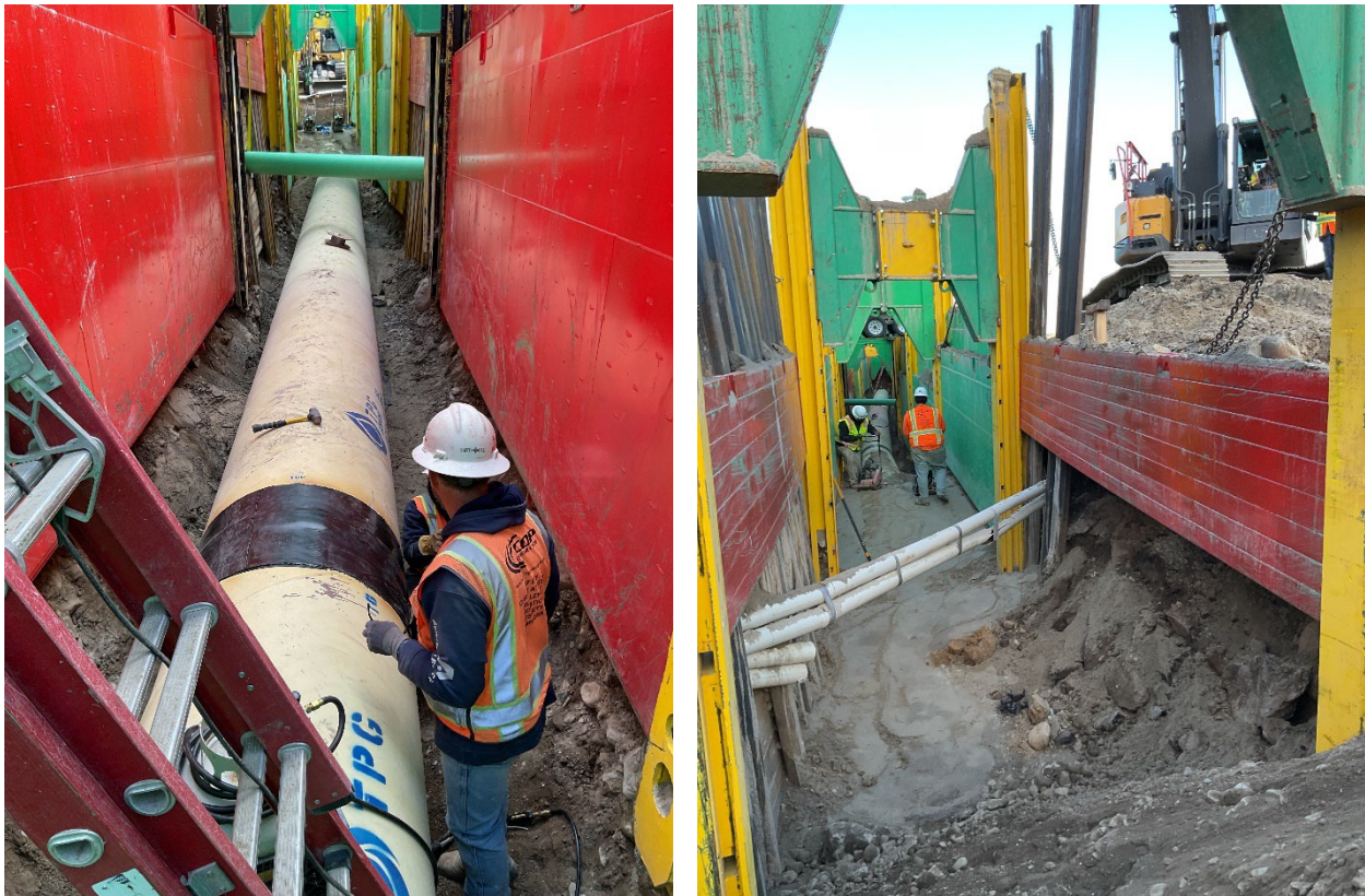
October 31: The contractor worked around collapsible materials along the CC-1 alignment.
