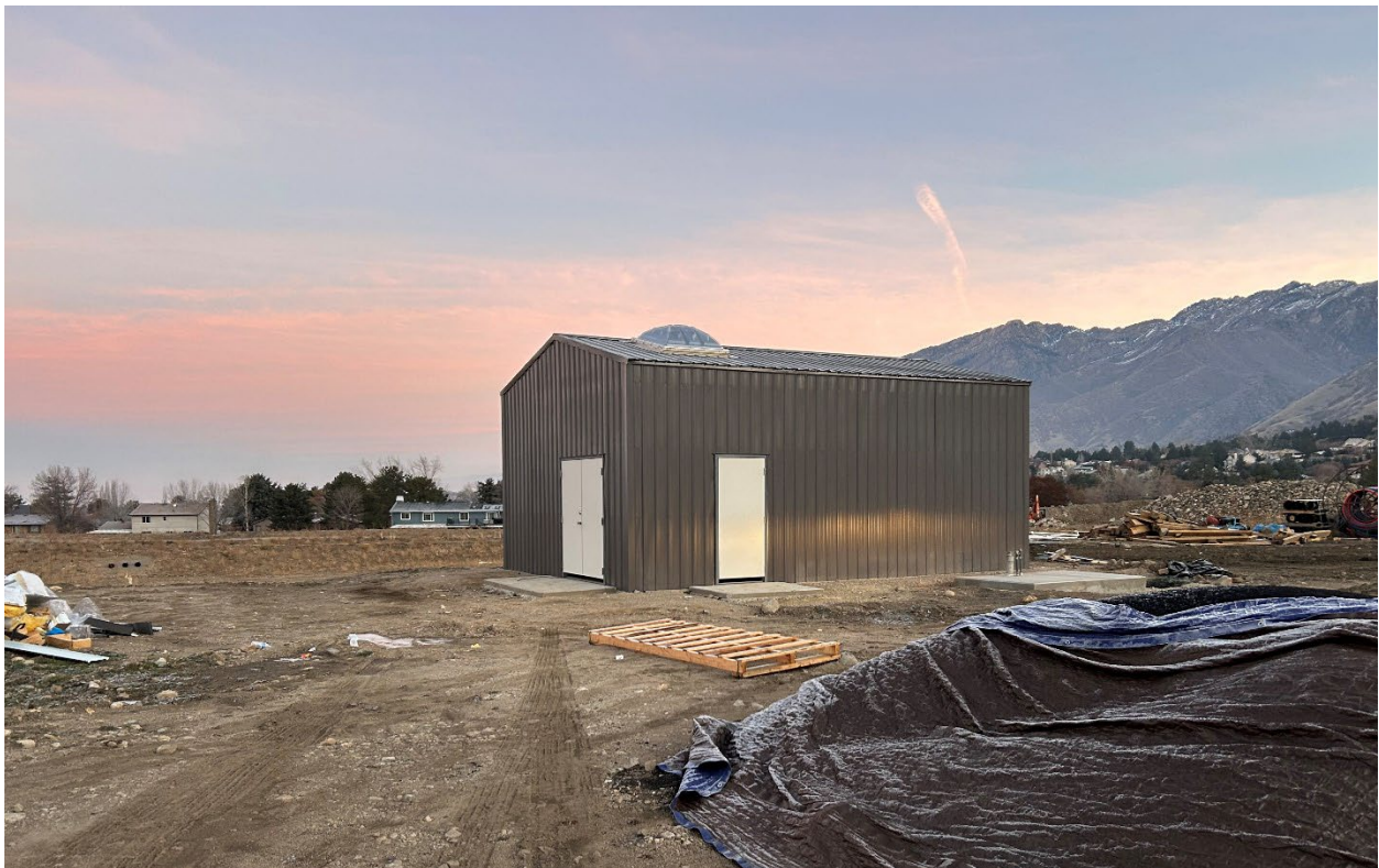
December 2: The MAR well house is constructed, albeit with temporary doors.
