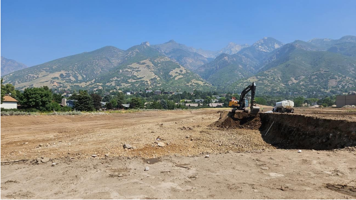
Aug 30: Excavation on the north surface infiltration basin.
