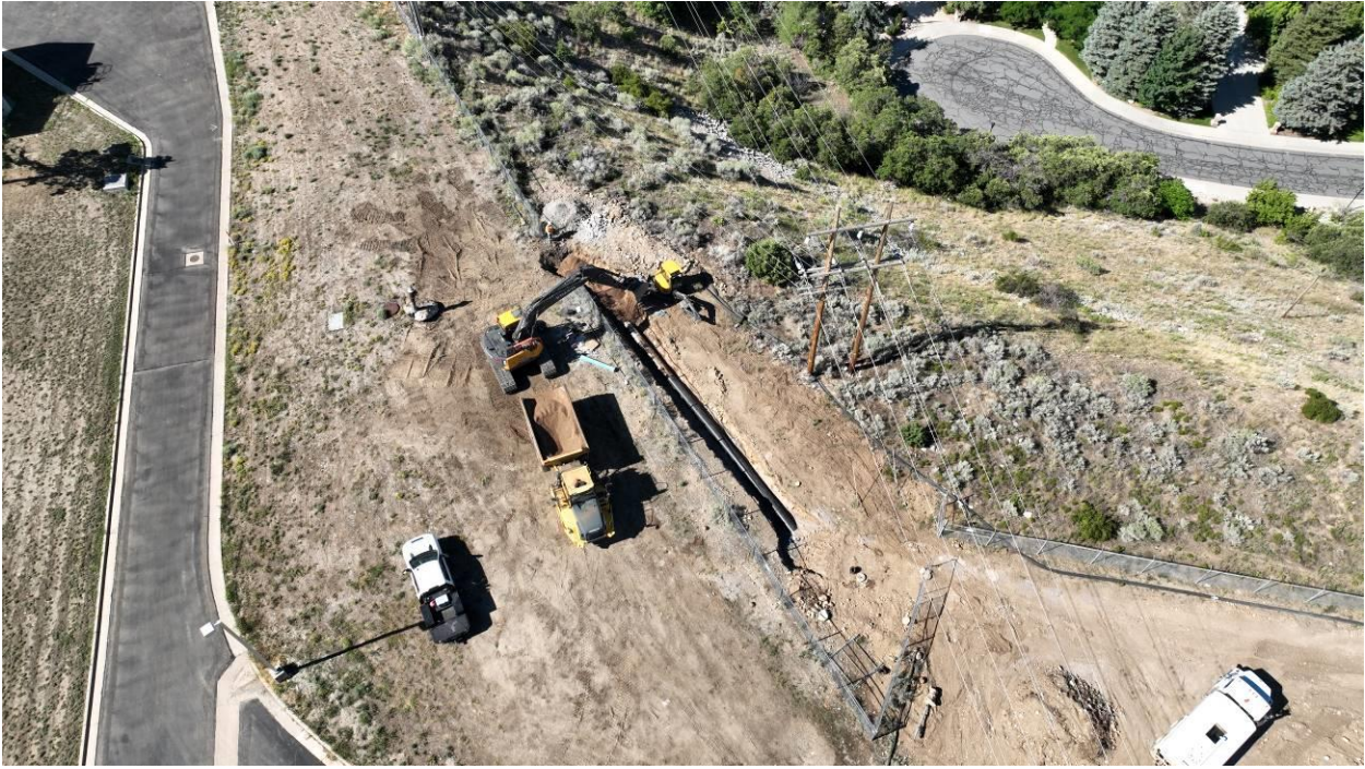
Aug 29: Southwest tie-in to existing ASR piping.
