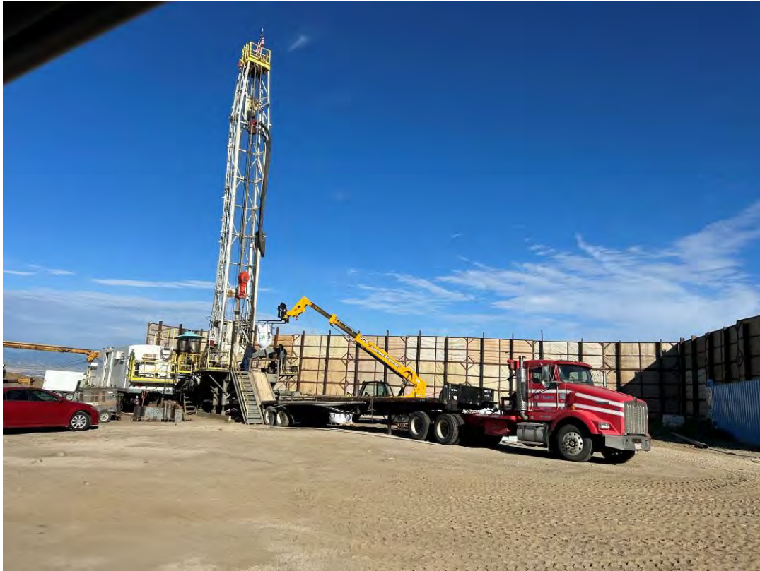
September 13: The gravel pack was installed around the ASR well.
