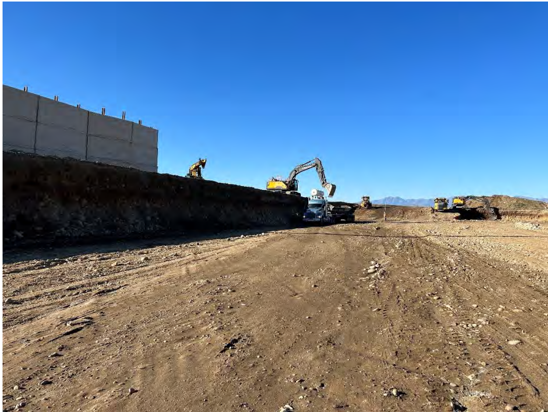
September 26: Excavation on the south surface infiltration basin.
