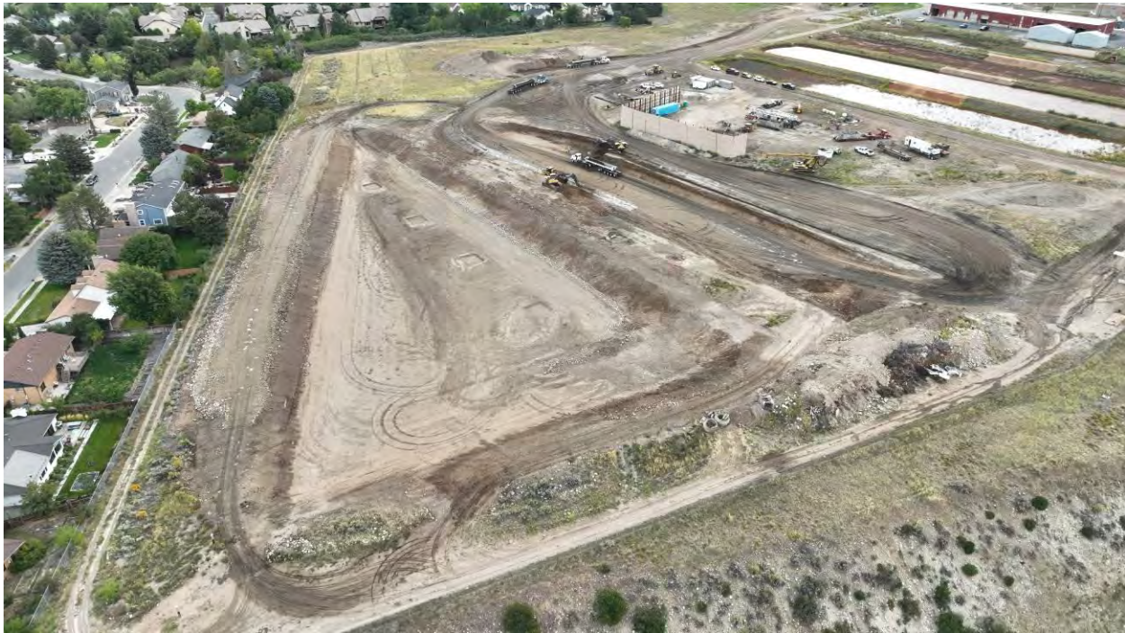
September 20: Overall site progress.
