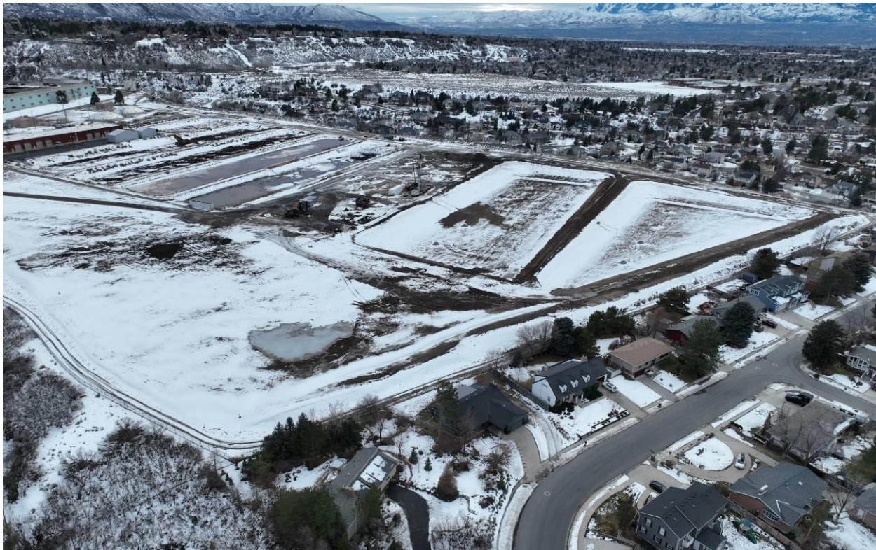
January 22, 2024: Overall site progress.
