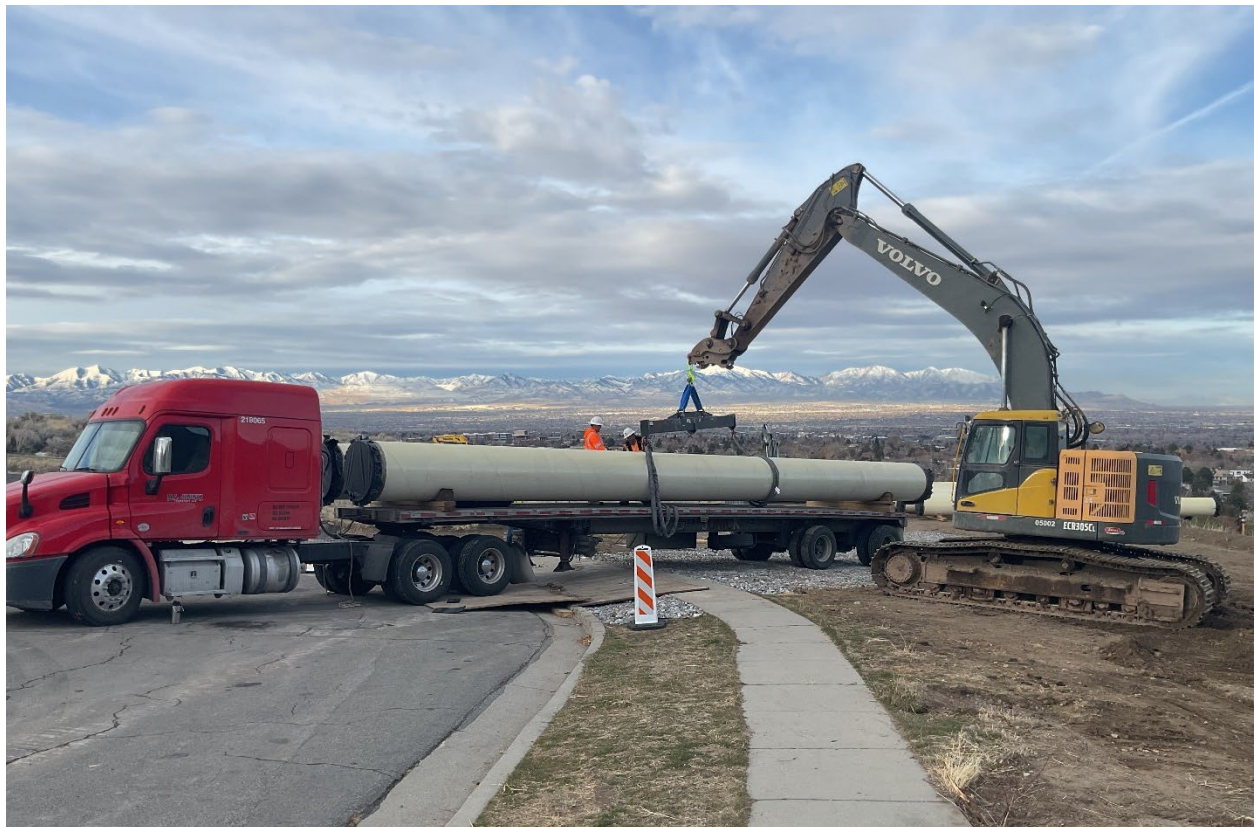
December 16: The contractor received 36-inch diameter pipe for the LCC relocation.
