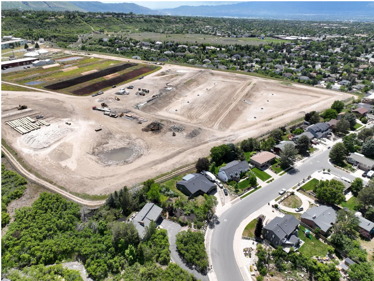
May 28, 2024: Overall site progress.
