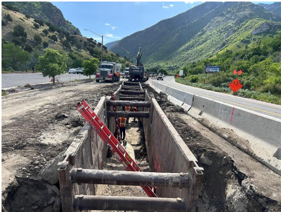
May 29, 2024: Pipe construction on Big Cottonwood Road east of Wasatch Boulevard.
