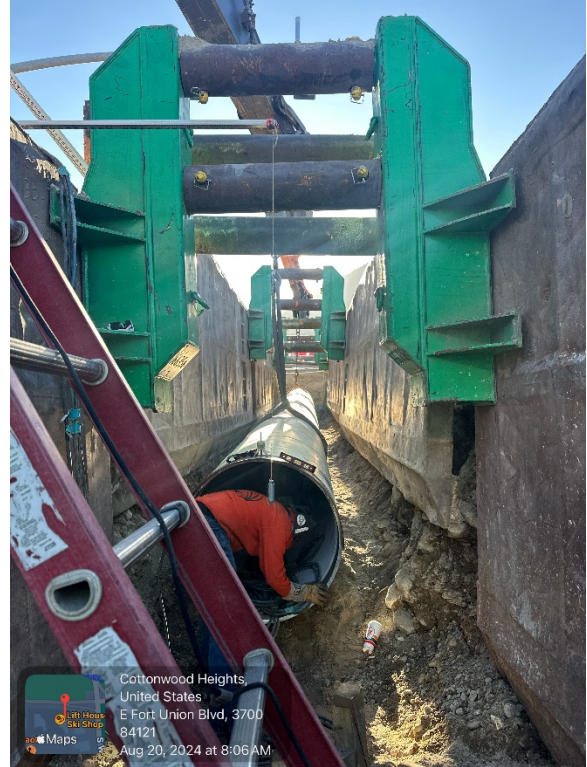
August 20: Welders enter the 36" diameter pipe to weld joints between each 50' length.
