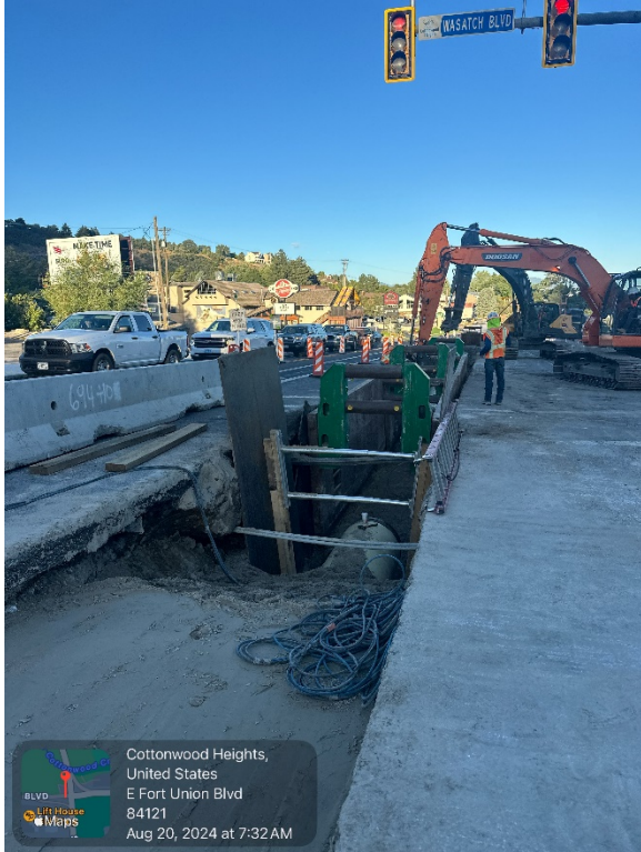
August 20: Welders enter the 36" diameter pipe to weld joints between each 50' length.
