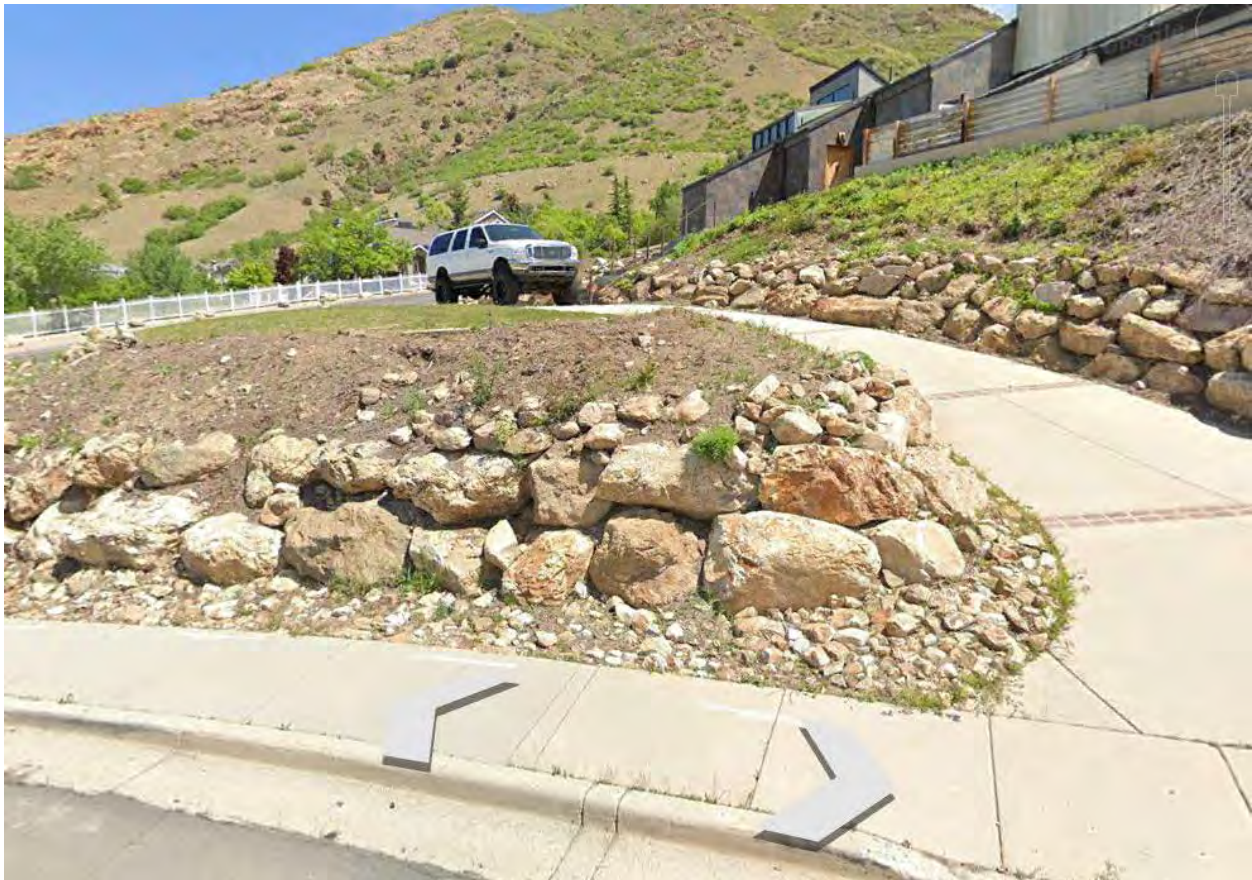
Original Driveway and Rock Walls (Google Earth, September 2021). Looking North.
