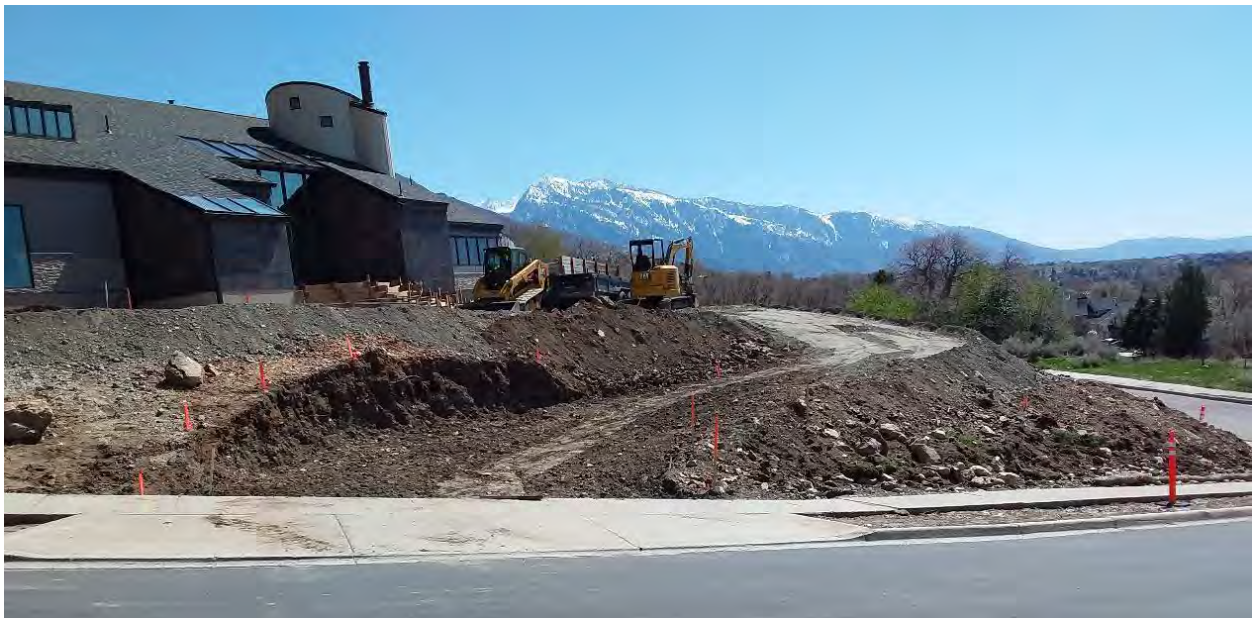
Earthwork (April 2022). Looking South.
