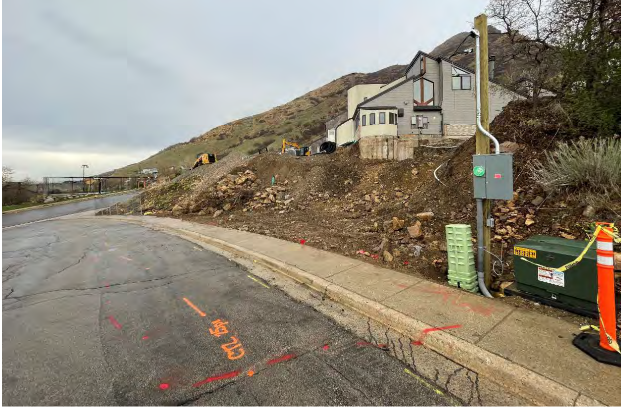
Earthwork (April 2023). Looking North.
