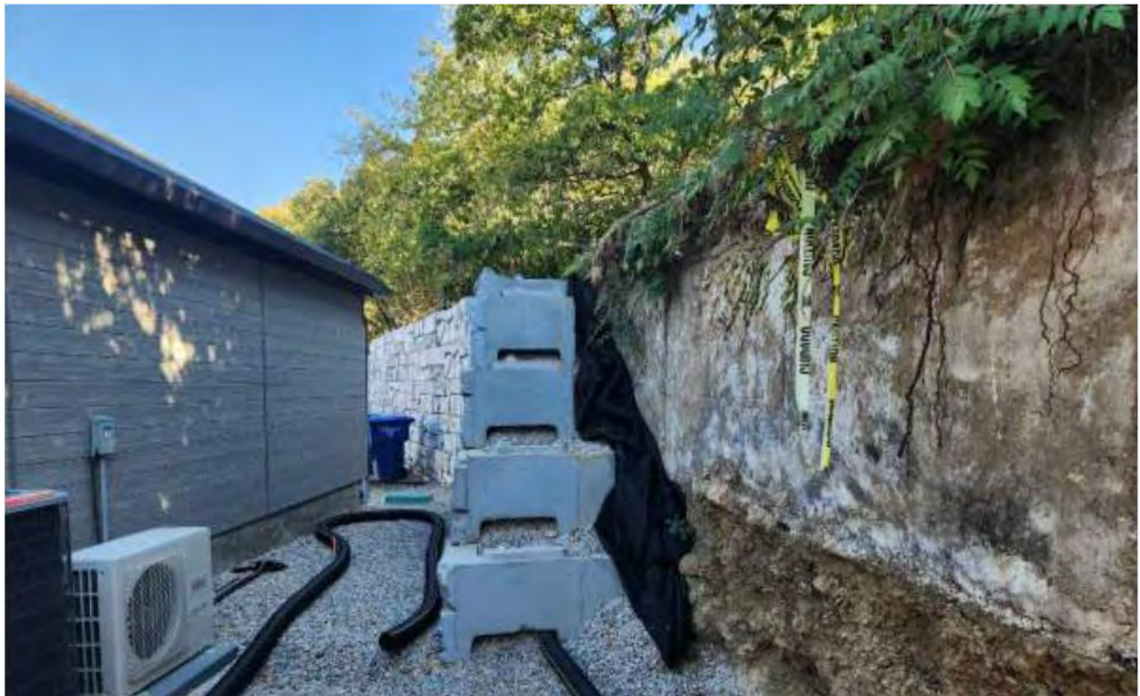
Applicant Verti-Block Wall (East of Home).
